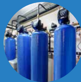
RETROFIT & REVAMP OF EXISTING TREATMENT PLANT
